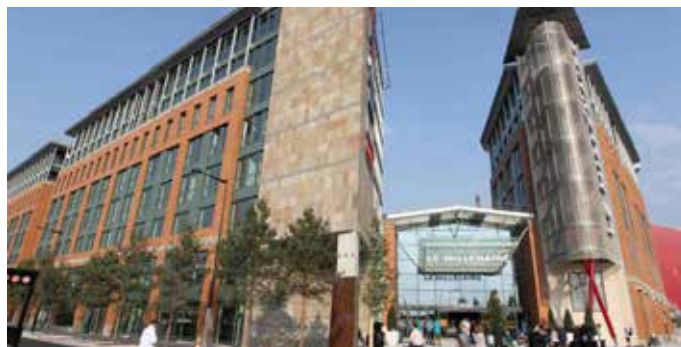
Partitions and doors - «Le Millénaire» shopping centre Aubervilliers, France
