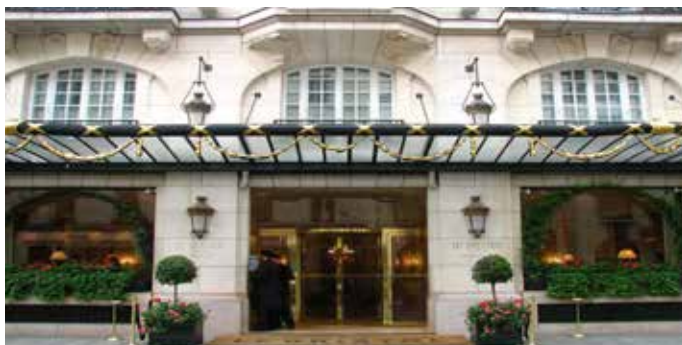
Phonic insulation - Bristol Hotel Paris, France
